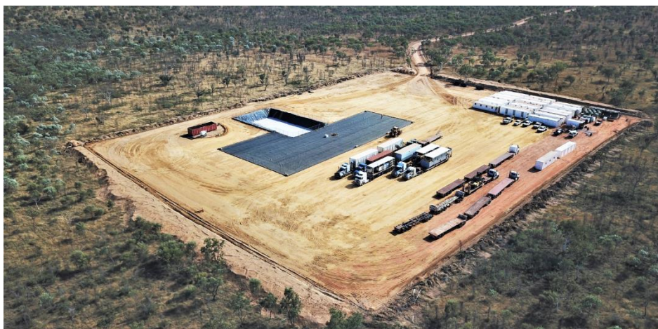
Rig trucks unloading at the Currajong well site
