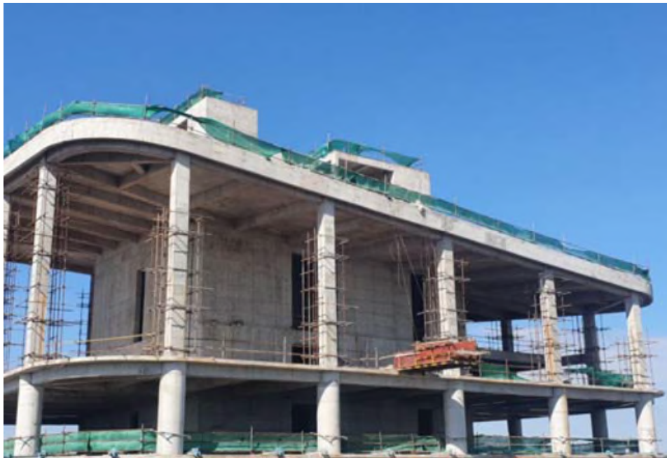
Figure 4: Tower 1 – Roof Top
