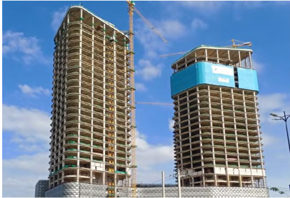
Figure 3: Overall view of Tower 2 and Tower 1
