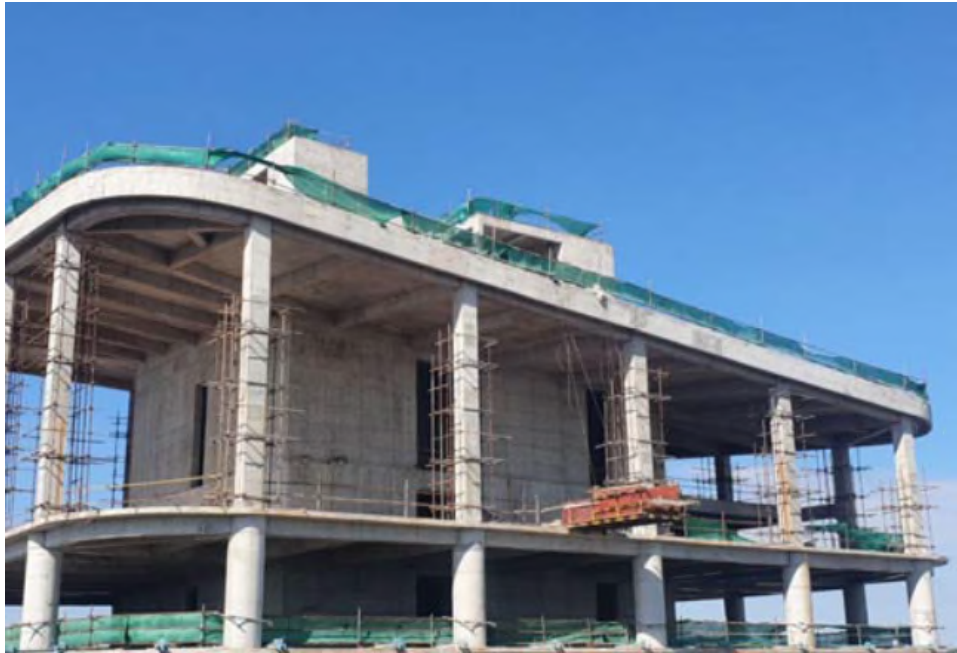
Figure 4: Tower 1 – Roof Top
