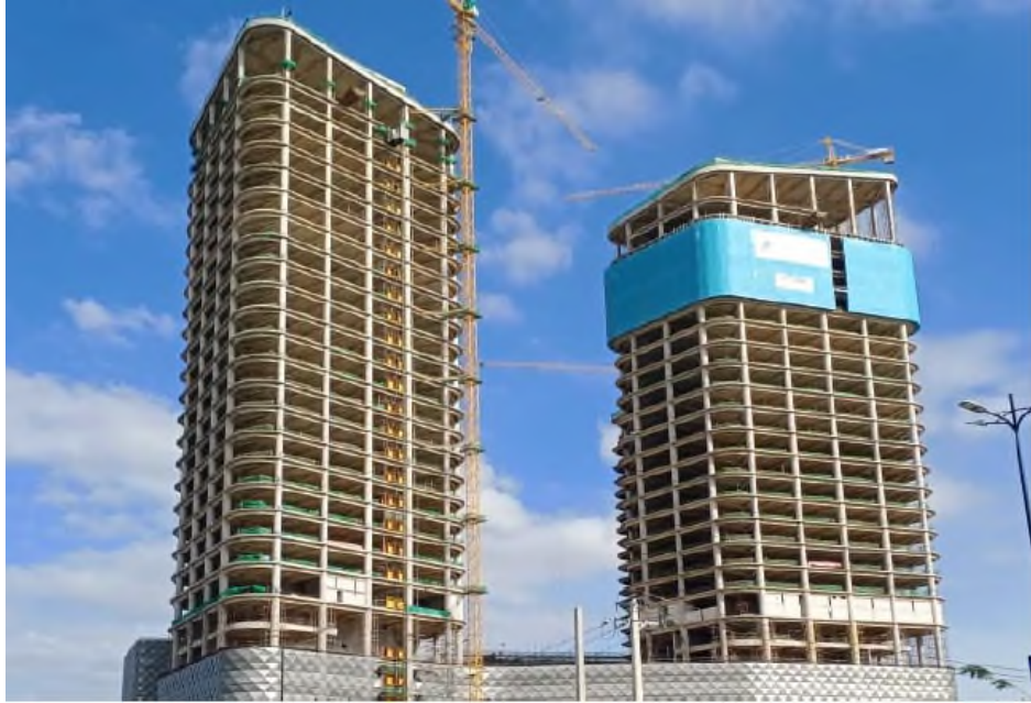
Figure 3: Overall view of Tower 2 and Tower 1
