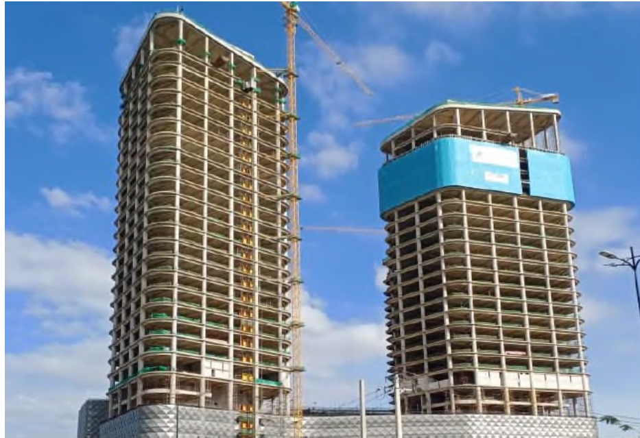
Figure 3: Overall view of Tower 2 and Tower 1
