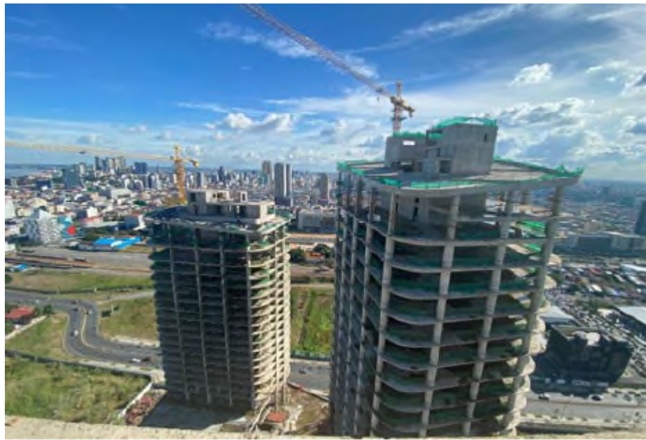
Figure 2: Overall view of Tower 2 and Tower 1
