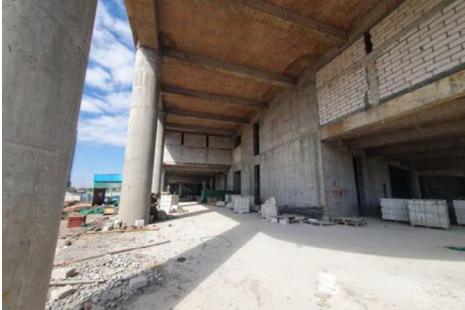
Figure 5: Tower 2 – Ground Floor – Overview of Main Lobby
