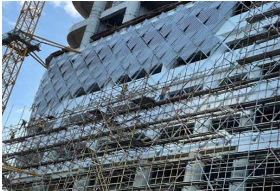
Figure 6: Tower 2 – Level 5 to Level 7 – Installation Aluminium Perforated Façade Panel
