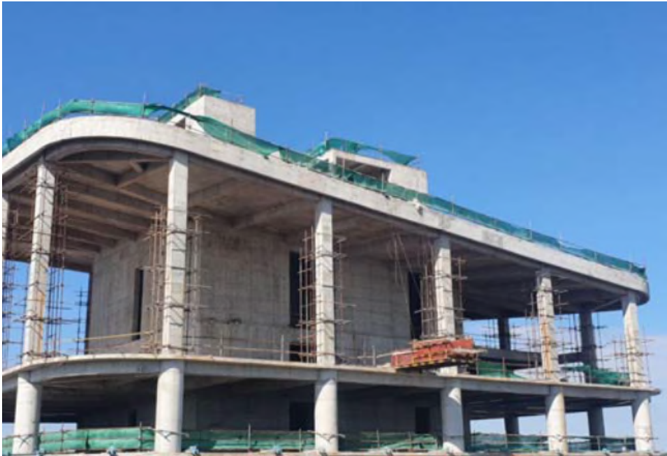
Figure 4: Tower 1 – Roof Top
