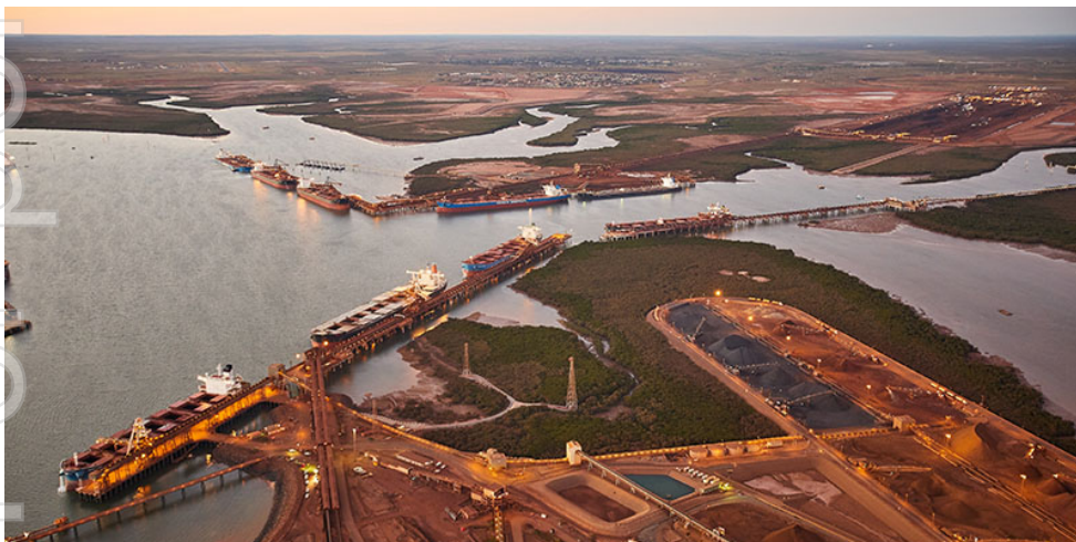
Utah Point bulk loading facility: Photo courtesy of Pilbara Ports Authority.
