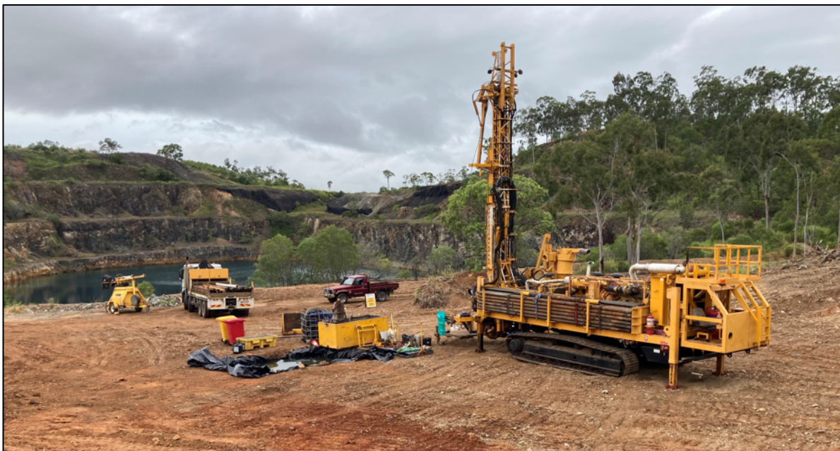
Figure 3: DDH1 Drilling multipurpose UDR 650 rig onsite at the Mt Chalmers Copper Project.
