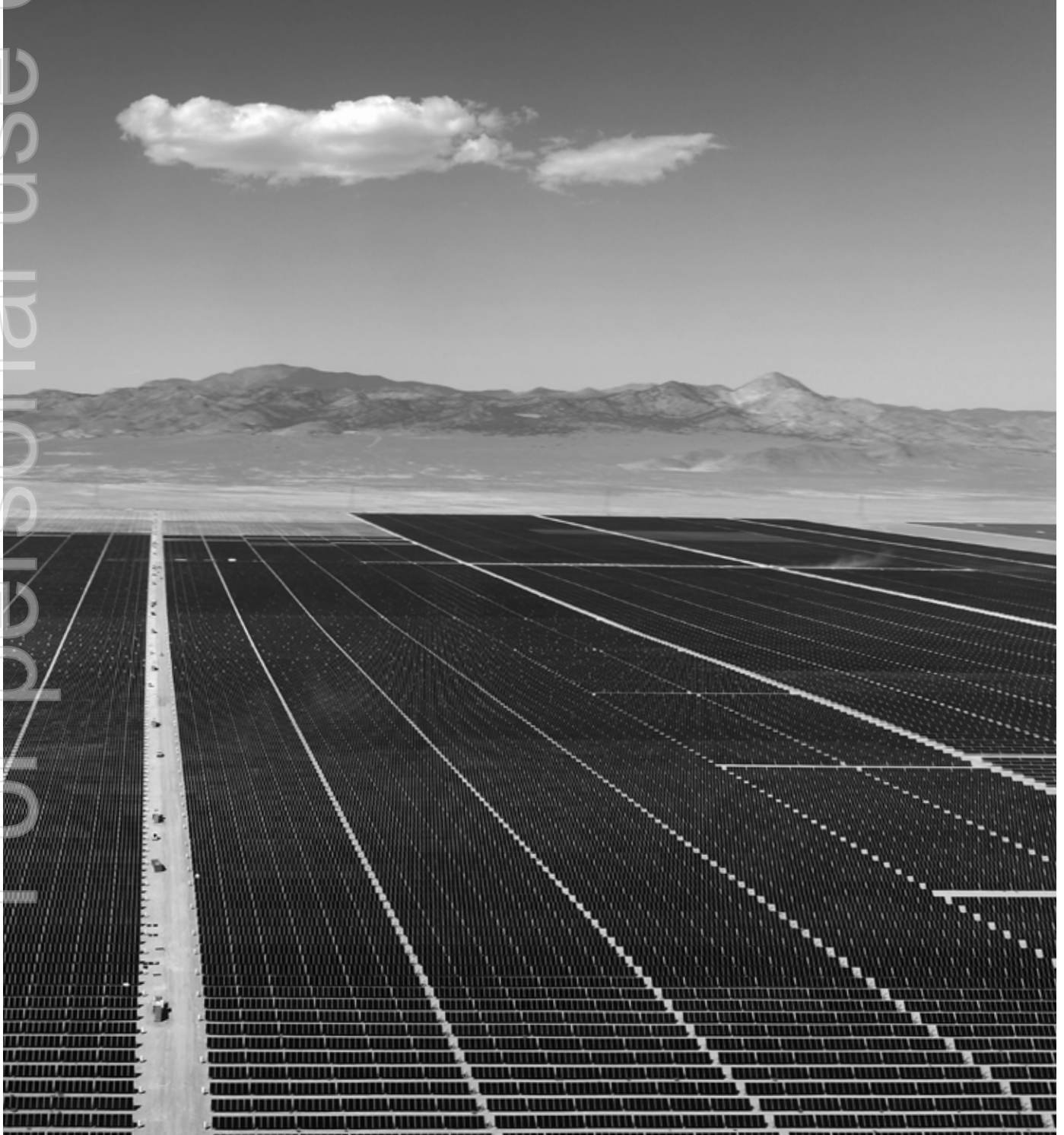
Prospero Solar project, Texas, USA.
