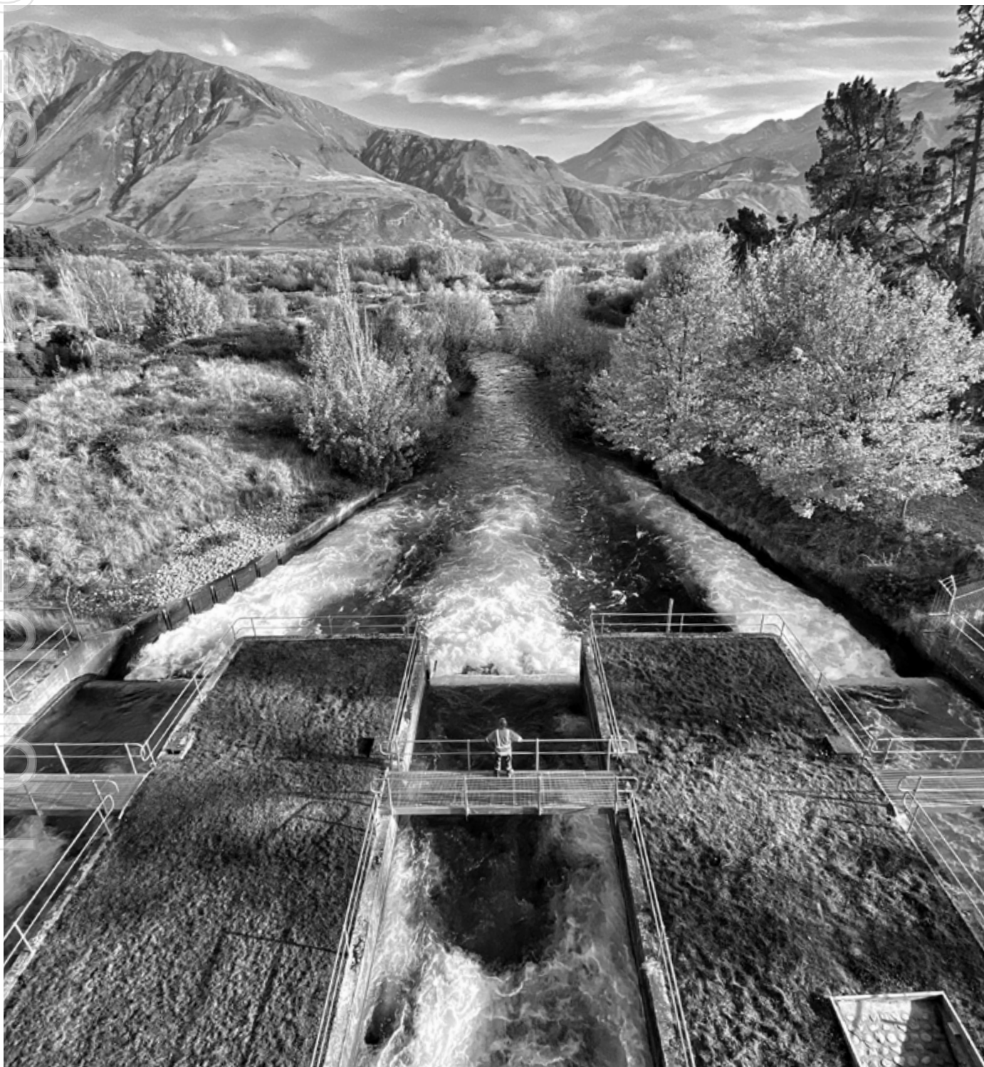
Lake Coleridge Power Station
