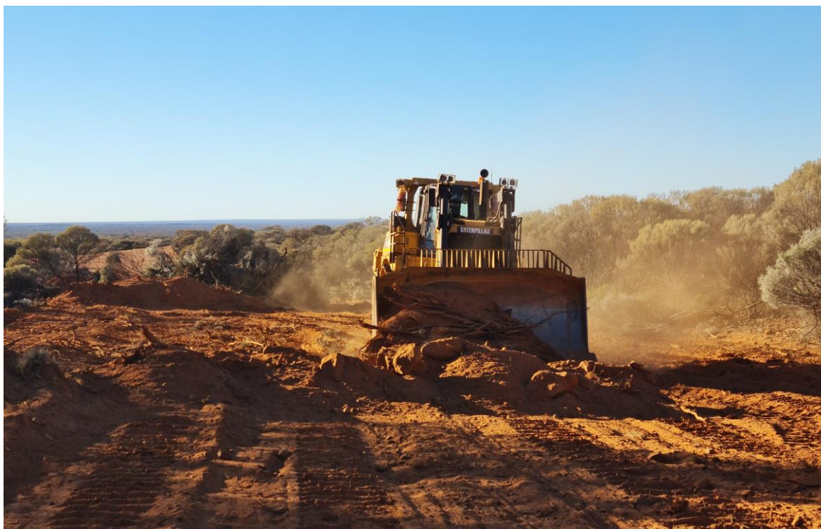
Image 1- Haul road construction
