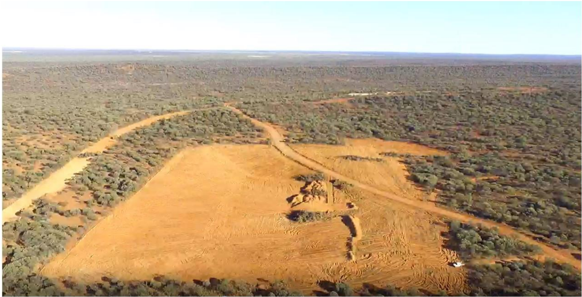
Image 2 – ROM Ore Pad, Plant site, Production Stockpile location - under construction
