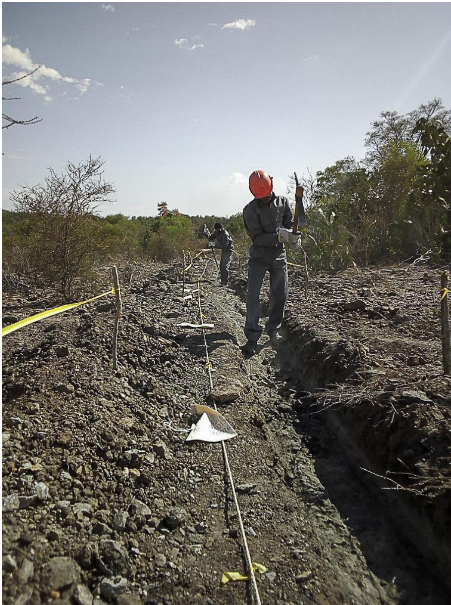
Figure 1 - Trenching continues in the Northwest Razafy Area
