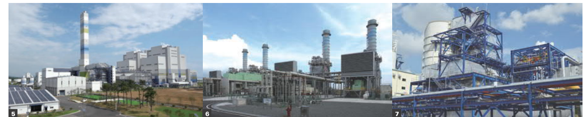
7 O Mon 330MW Oil & Gas Power Plant, Vietnam [ SEP 2012 - NOV 2015 ] Daelim Industrial's first EPC on Oil & Gas thermal power plant
