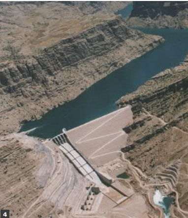
3 Busan New Port Phase 1, South Korea [ JAN 2001 – MAY 2009 ] Logistics base terminal for Northeast Asia (Wall extension: 3.2km) 4 Karun Dam, Iran [ DEC 1994 – APR 2001 ] Large-scale rock-fill dam / 228 million tons storage / 250MW x 8 5 Hantan River Dam, South Korea [ FEB 2007 – DEC 2016 ] Large-scale flood control dam (RCD method) / (H)83.5m x (L)690.0m
