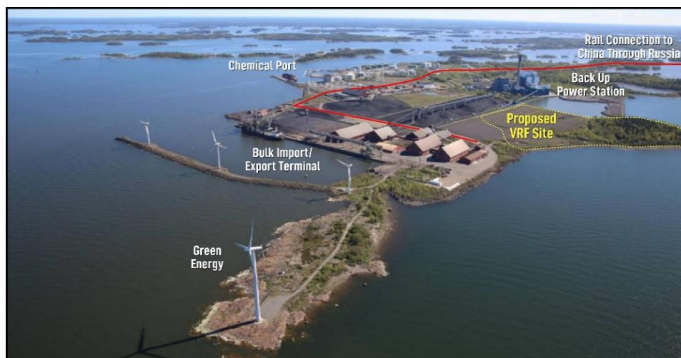
Figure 2 - Aerial schematic showing location for the proposed Vanadium Recovery Project processing plant at Tahkoluoto Port, Pori in Finland
