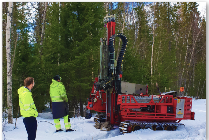
Geotechnical drilling at Talga's planned Anode Refinery site in Luleå.
