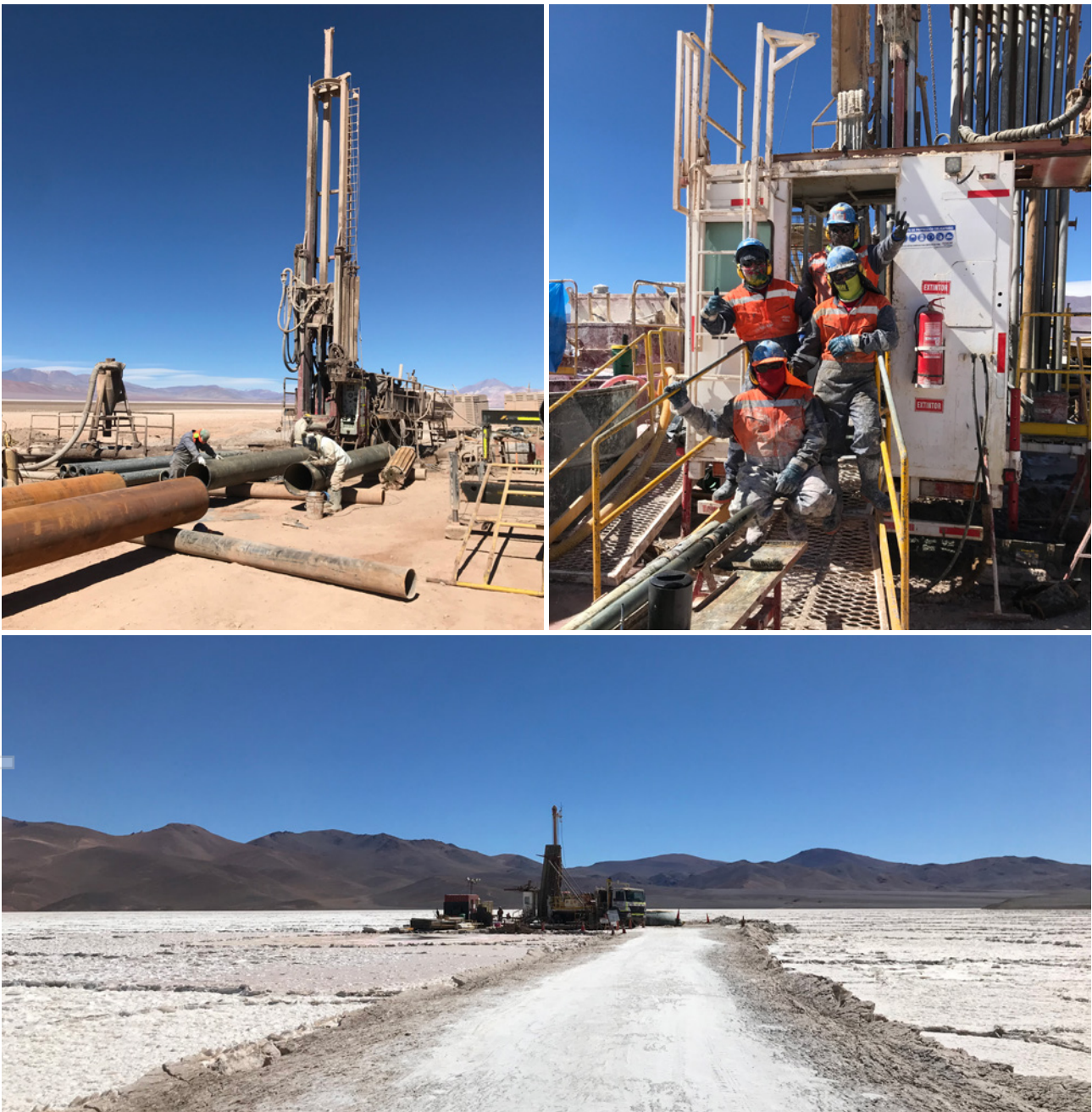
Figure 2: Contractor Andinor's construction of the 400m production well.
