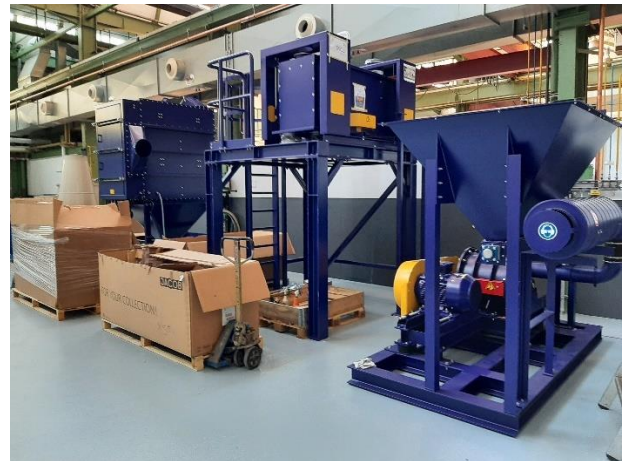
Figure 4 – DP Stage 1 Shredding and Sorting
