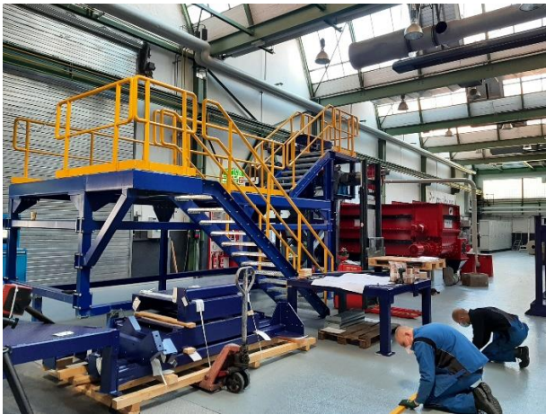
Figure 3 – DP construction activities in Hilchenbach
