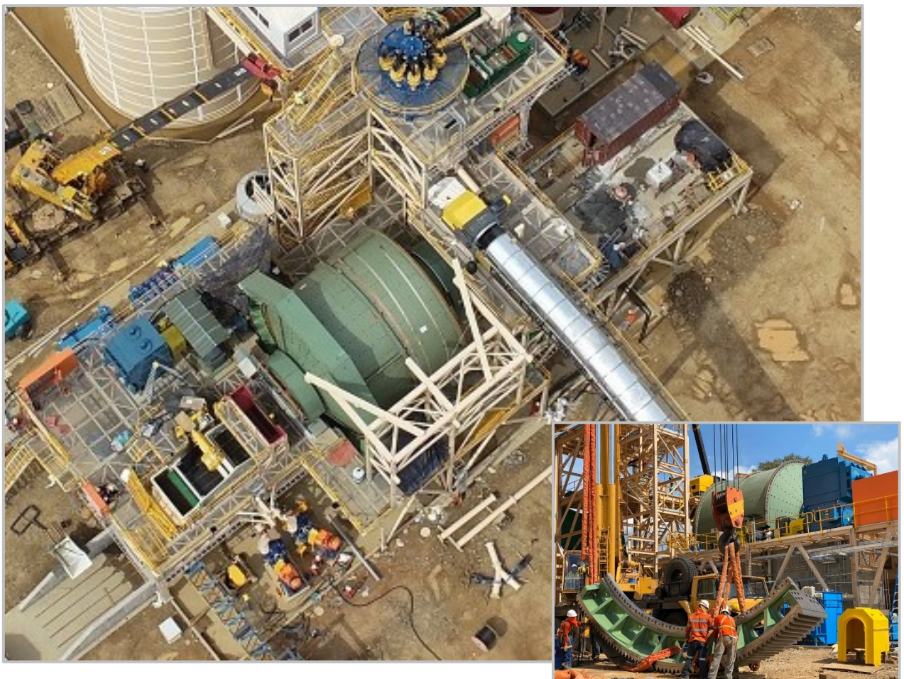
Figure 3 | SAG Mill installation nearing completion
