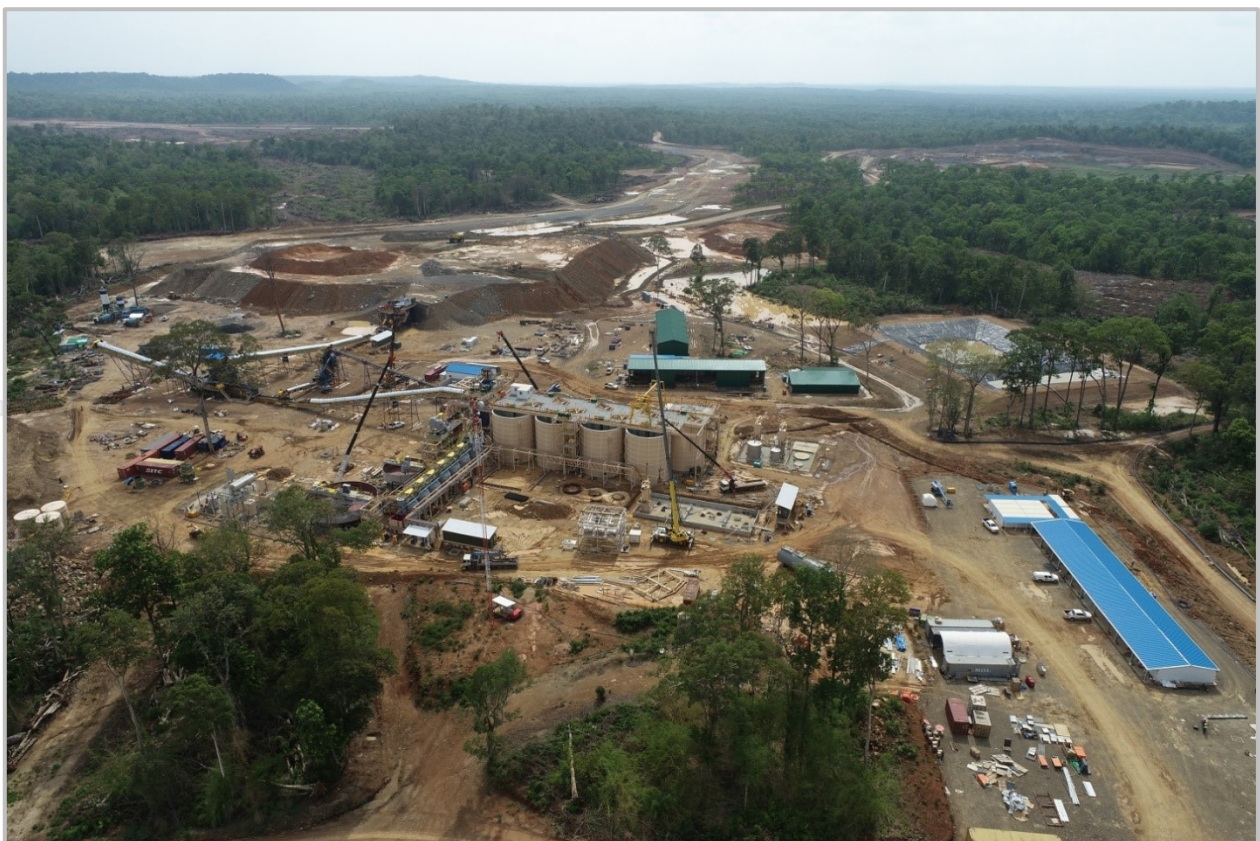
Figure 1 | Okvau Gold Project Layout
