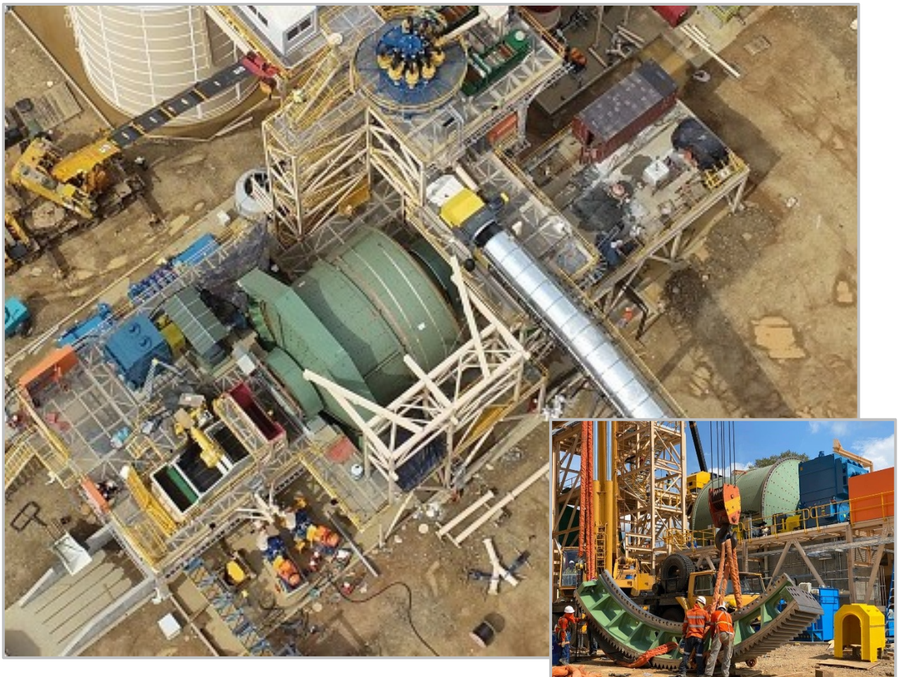
Figure 3 | SAG Mill installation nearing completion
