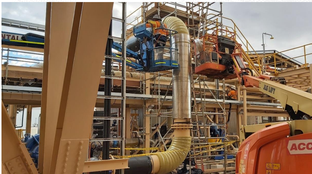
Figure 4: Installing thermal insulation to chilled water pipework
