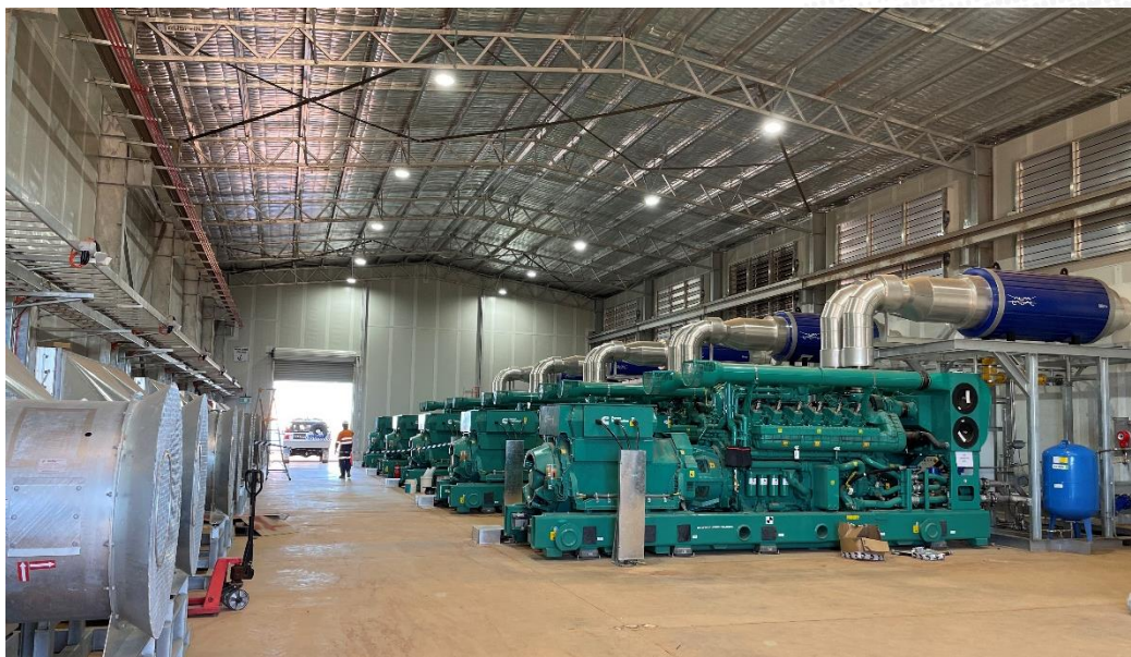
Figure 6: Five 2MW Cummins gas engines during commissioning
