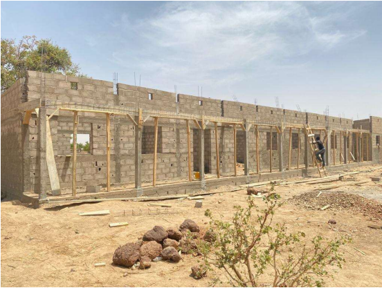
New school under construction by WAF.
