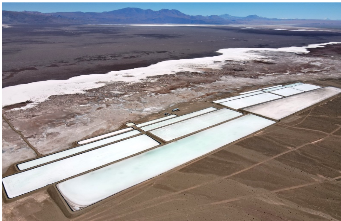
Figure 2. Rincon Lithium Project – 38Ha Operational Evaporation Ponds
