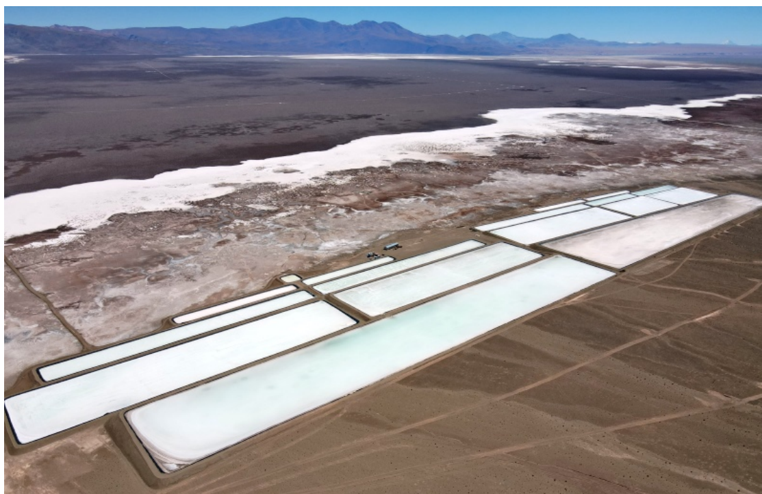
Figure 3. Rincon Lithium Project – 38Ha Operational Evaporation Ponds
