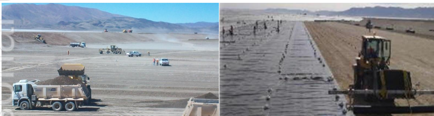
Note: additional ponds under construction
