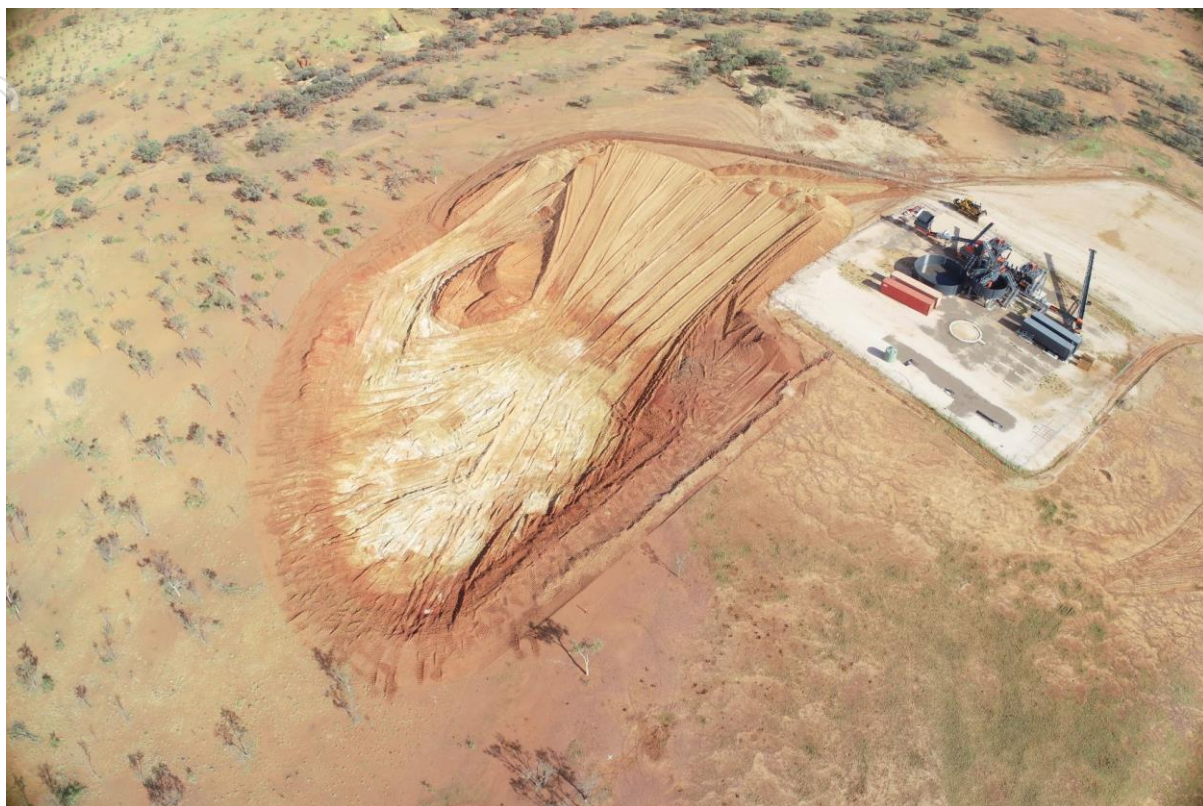
Photo 1 – Ardmore Pit excavation close to process plant
