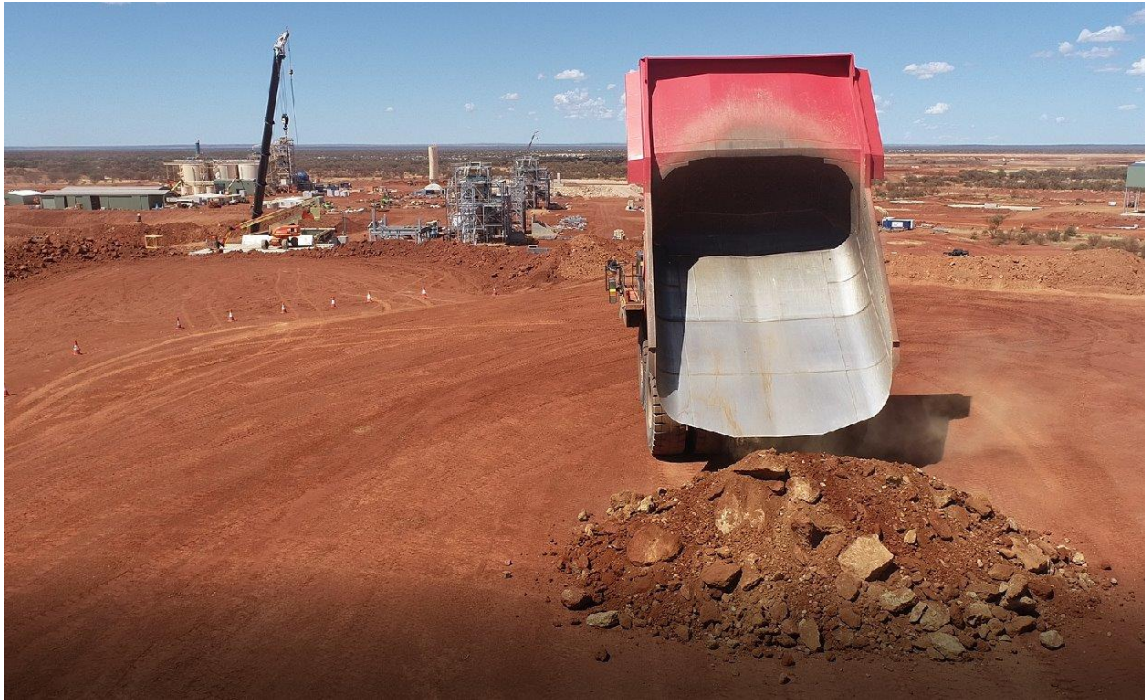
First load of ore to the ROM pad
