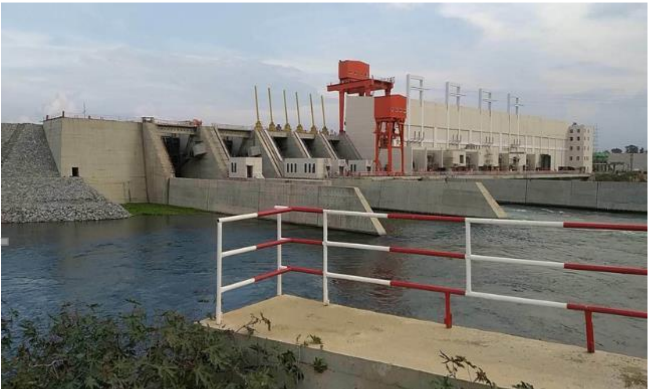
Figure 1: 183 MW Isimba hydroelectric power station.
