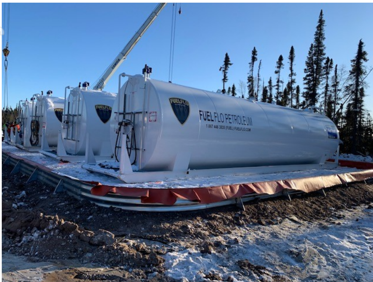
Figure 5: Completion of the installation of the fuel farm to service mining operations
