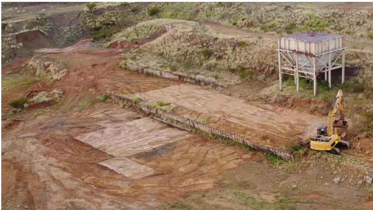
Figure 12: Exposing the original CIP concrete slabs, Mt Freda, next to Leach Vats Gold Processing.
