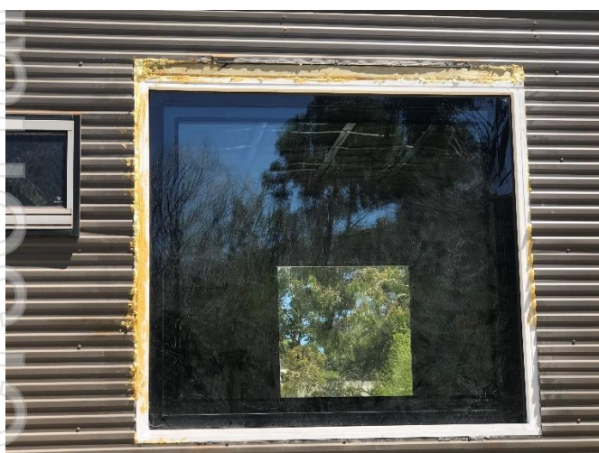
ATCO mining hut being retrofitted with ClearVue PV IGUs and Mirreco's Hemp panel insulation – view is through the installed IGU panels.
