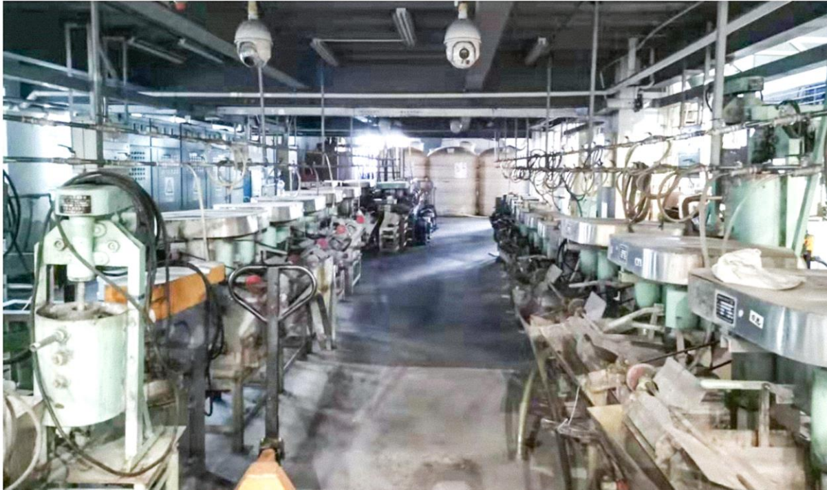
BGRIMM's large scale graphite pilot plant
