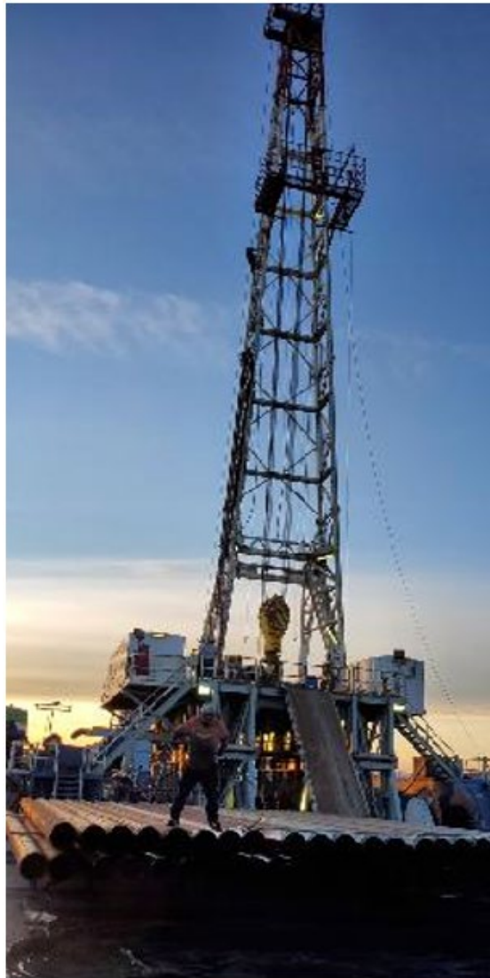
Graham Drilling Rig 5 at Borba 1-7
