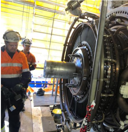
One of the four gas turbines disassembled during the overhaul
