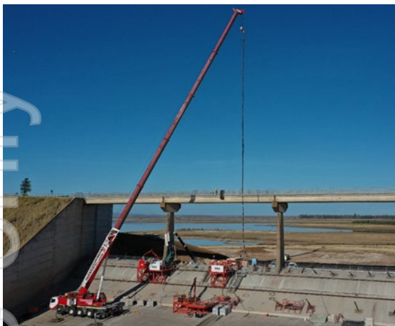
Fairbairn Dam Sunwater, Queensland Specialist Dam Anchoring “Water Infrastructure”
