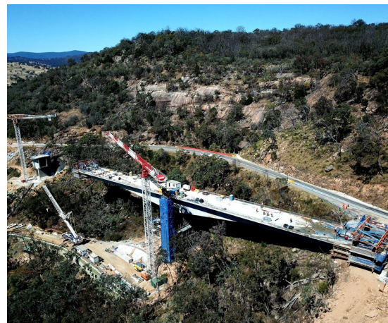
Bolivia Hill Transport for NSW Specialist Bridge Construction “Transport Infrastructure”
