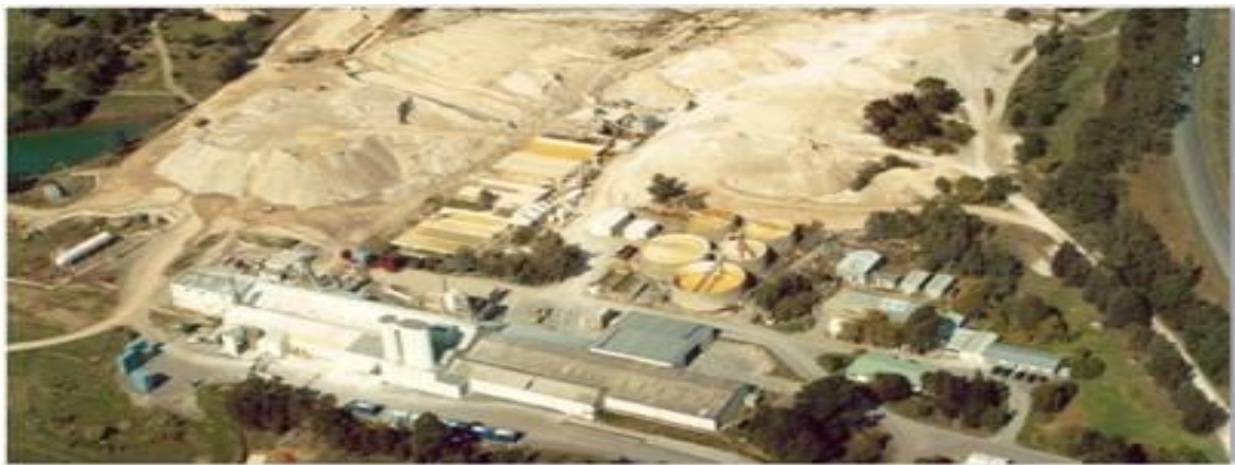
Pittong processing plant facilities
