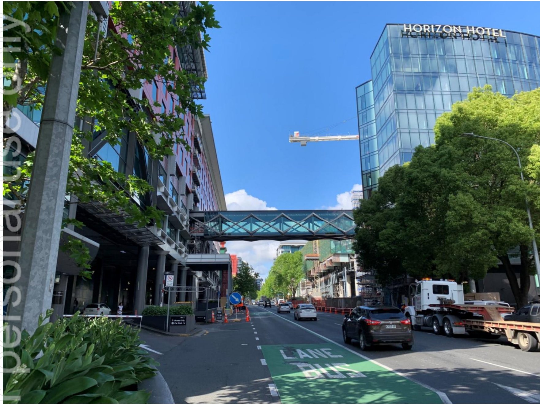
View from Hobson St – new linkway bridge
