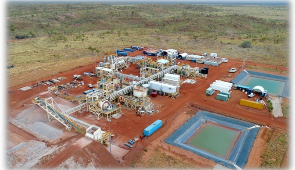
Browns Range Pilot Plant
