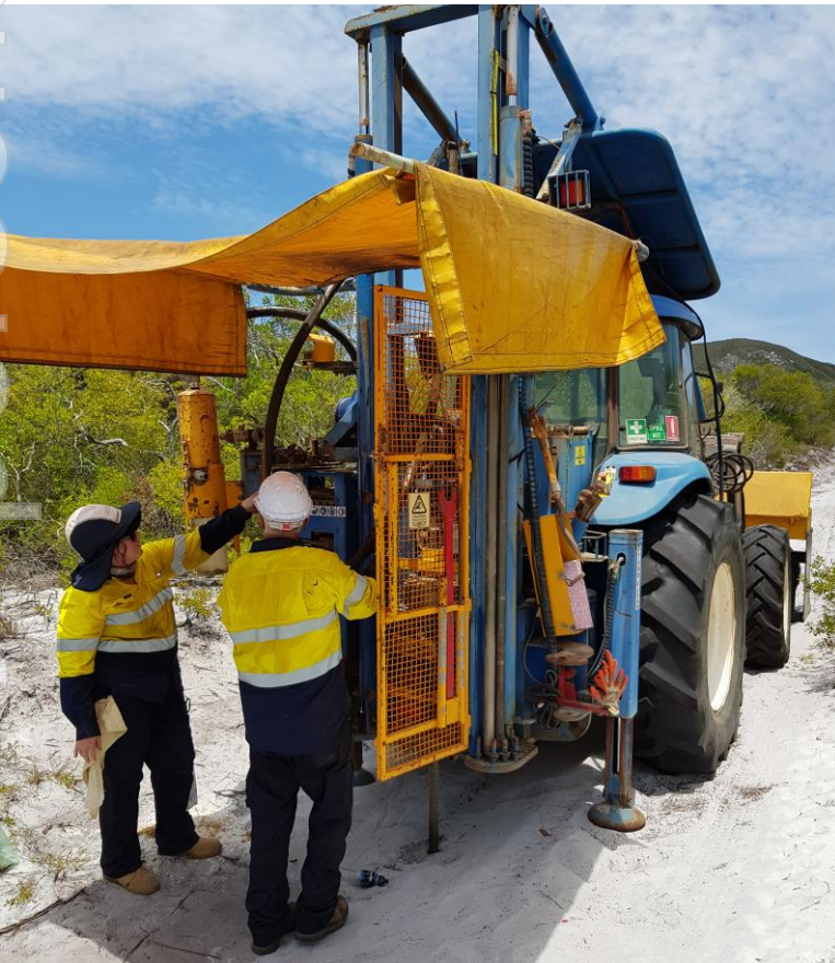
Yearlong Contracting Vacuum Drill rig
