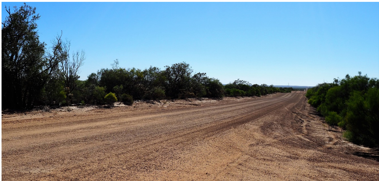
Mt Adams Road which Intersects the Beharra Tenement
