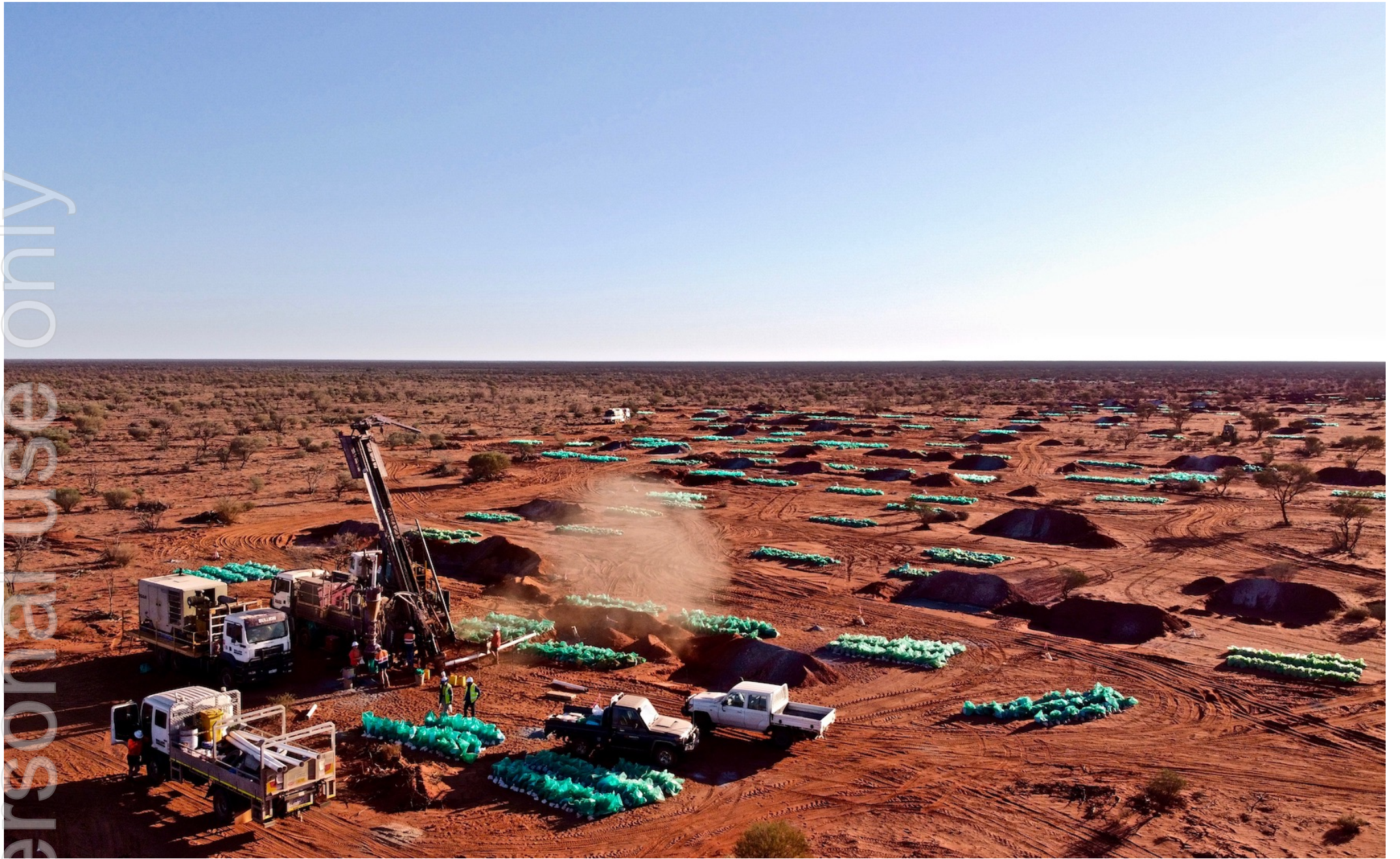
Figure 6: September 2020 drilling at Aurora Tank
