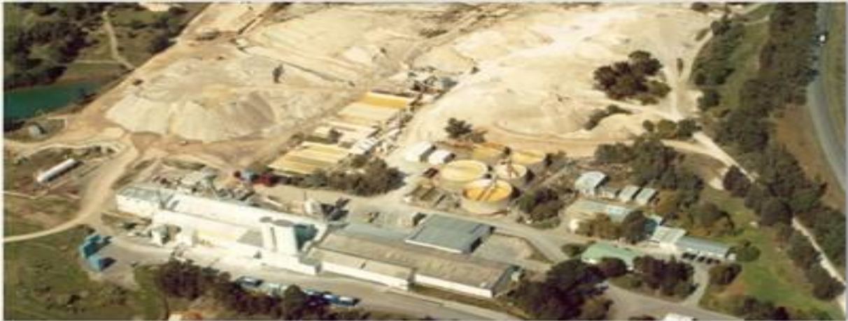
Pittong processing plant facilities
