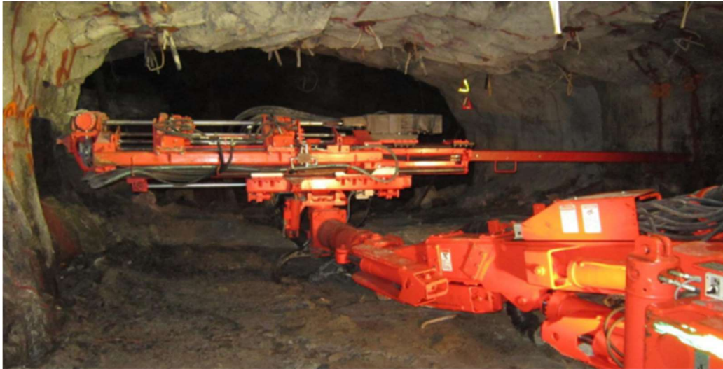
Figure 3: Sandvick Low Profile long-hole drill rig – operating from the on-reef drill drive
