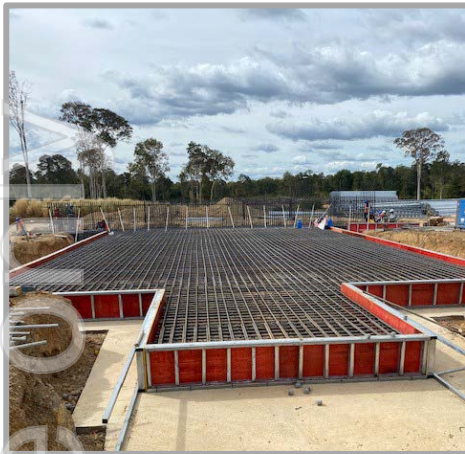
Figure Five | Primary Crusher Foundation Preparation
