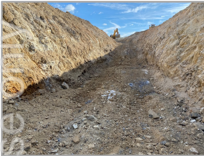
Figure Sixteen | Tailings Dam works & Keyway Excavation works
