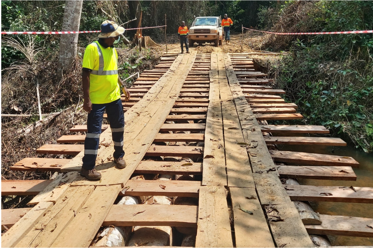
Figure 3: Access road building up at the Cestos gold project (Tietto 100%)
