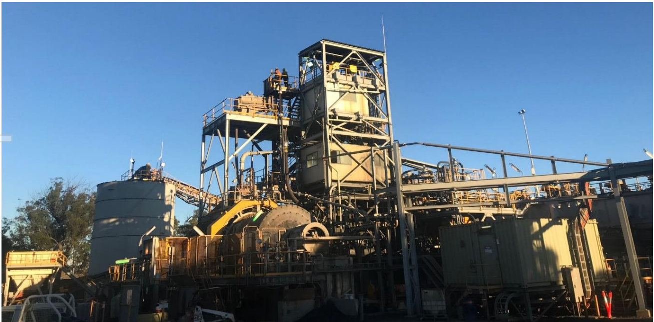
Figure 1 Hillgrove Processing Plant
