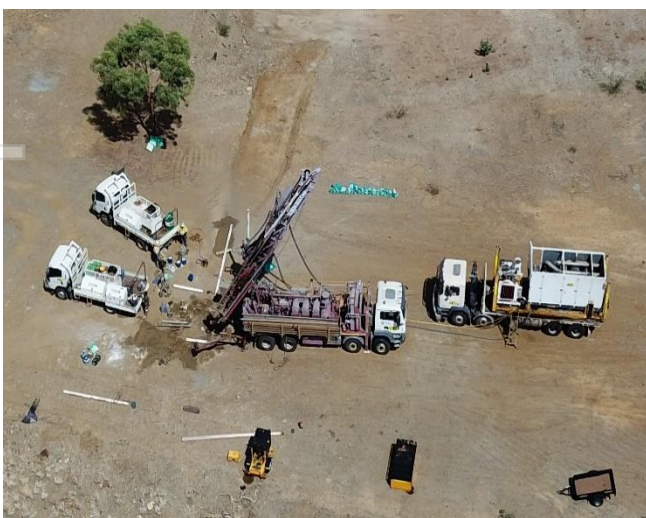
Photo 1. RC rig infill drilling at Mt Freda now completed.
