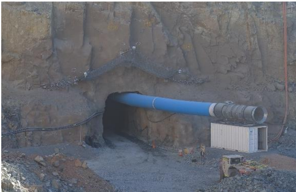
Figure 3: Deflector South West portal
