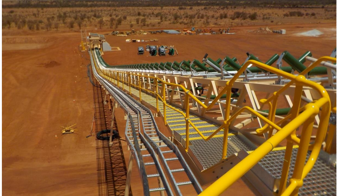
Figure 7: CV01 primary feed conveyor awaits belt fitting
