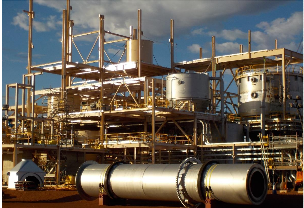
Figure 3: First tank installed onto 4 th floor and rotary drier awaiting install
