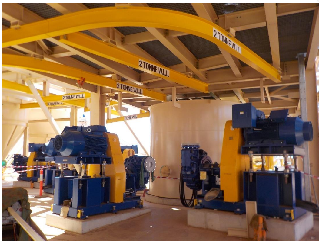
Figure 6: Brine recovery pond feed pumps 1-4
