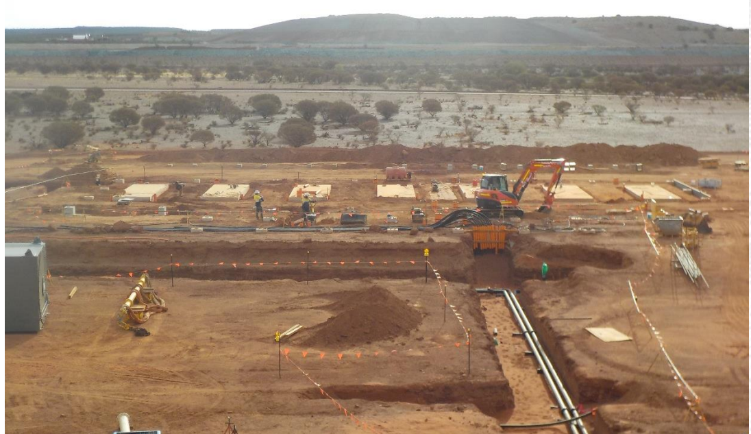
Figure 10: Concrete footings for 5x gas generator units and 2x additional footings for expansion activities
