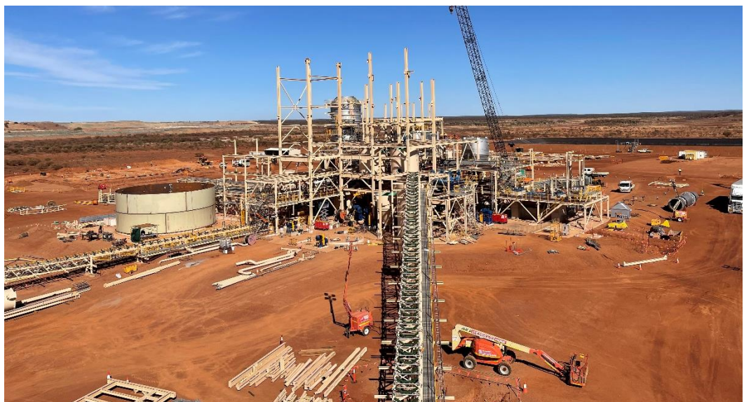
Figure 2: Process Plant structural steel erected to the 6 th floor
