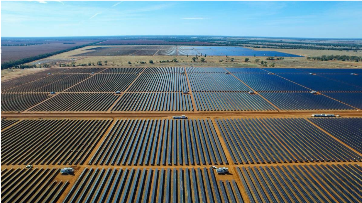
AGL's Nyngan Solar Farm, Central New South Wales
