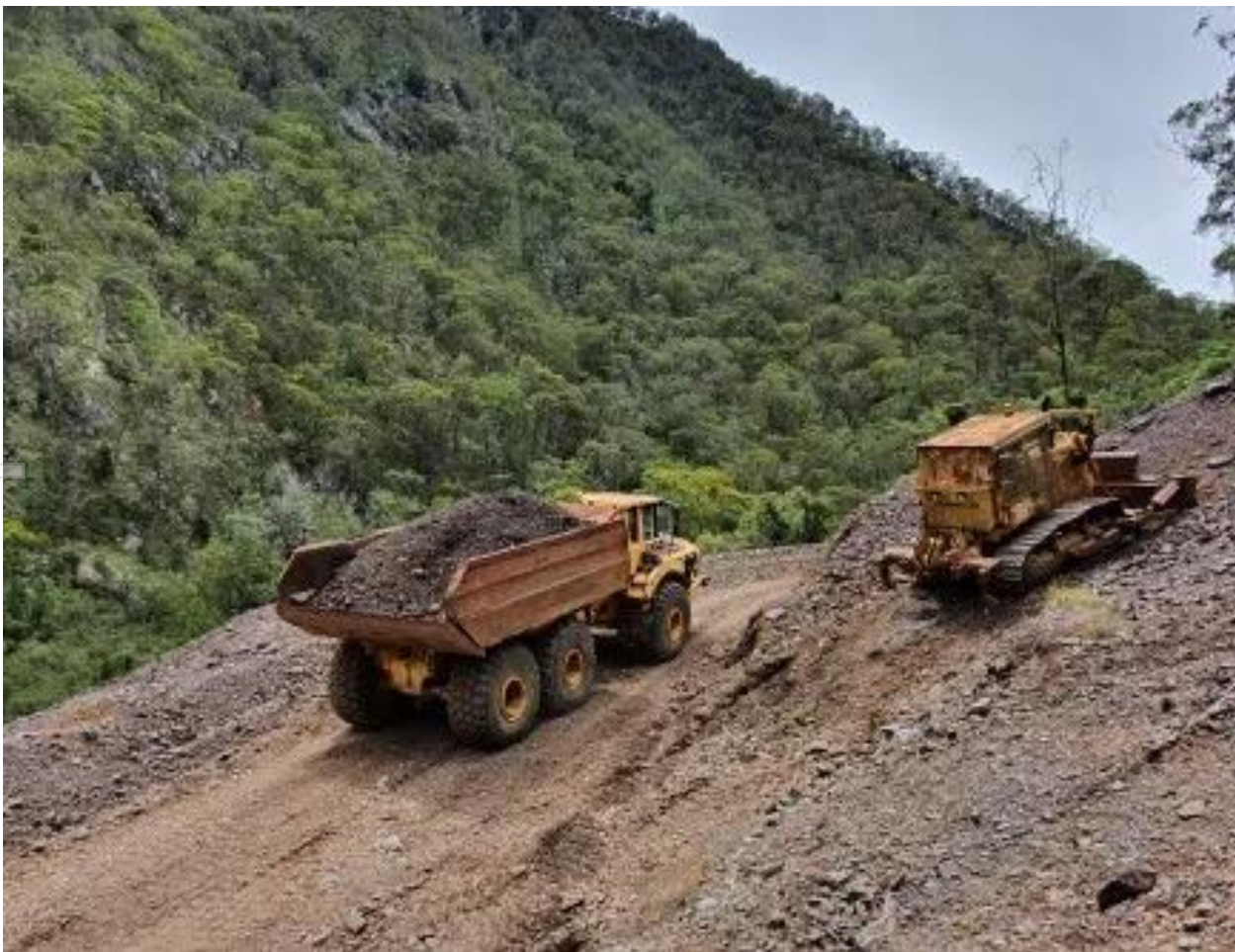
Figure 1 Bakers Creek Stockpile being hauled to Hillgrove Processing Plant
