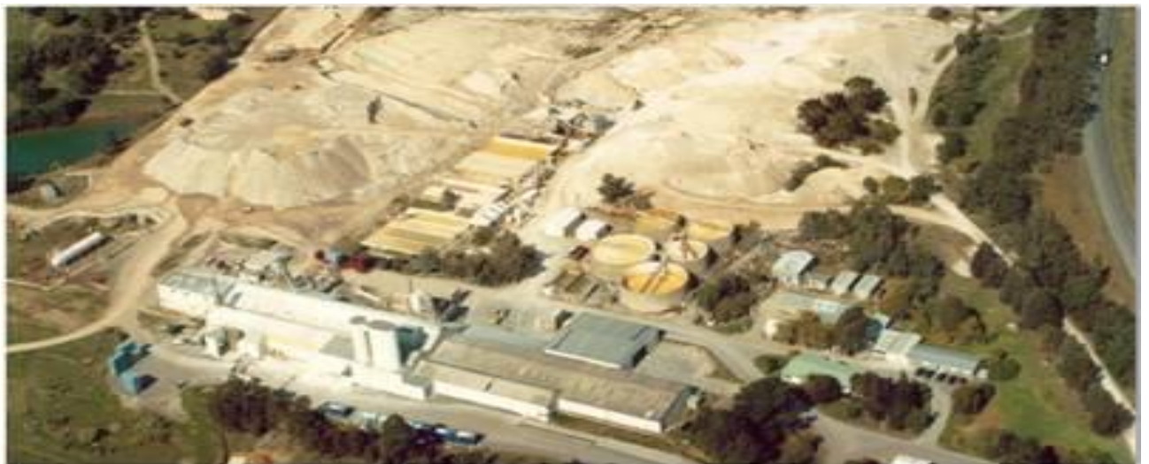
Figure 1: Pittong processing plant facilities
