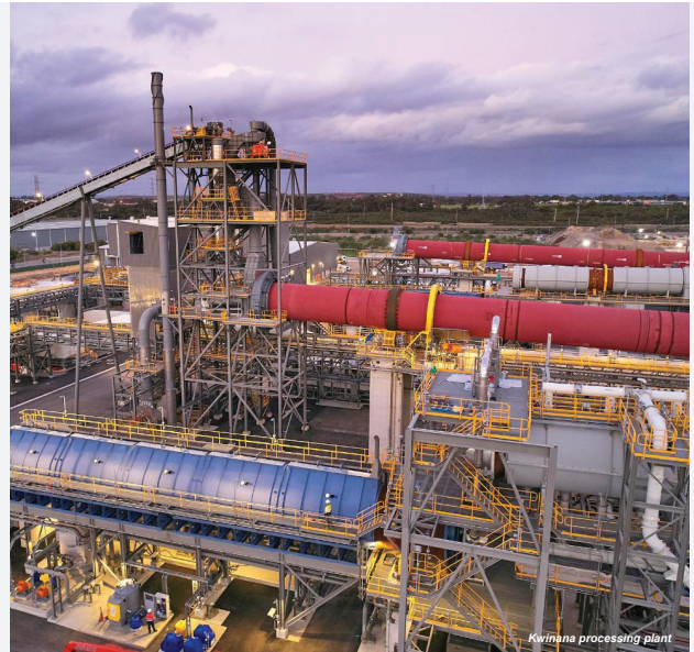
Kwinana processing plant
