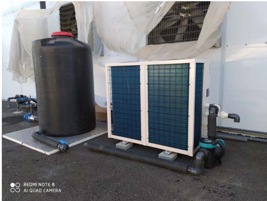
Image two: Water tank at My Green Fields cannabis farm to be used for temperature control
