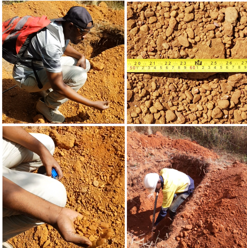
Photo 1. Screening and pitting activities
