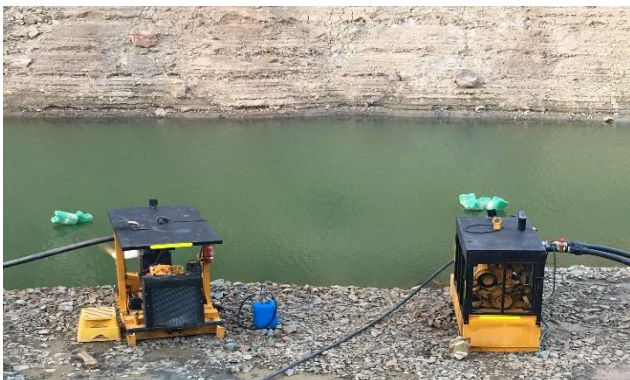
Photo 5. Pit dewatering pumps in action.
