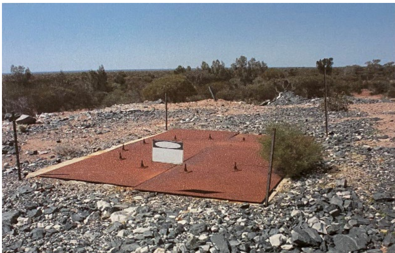
Vent rise - covered with steel plate
