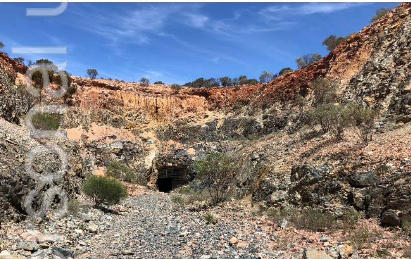
Boxcut to the decline at First Hit - access blocked and portal fenced
